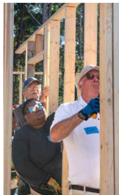
Vince Howe, above, nails top plate onto freshly raised wall section. Left: John Meyer, Dale Smith and a member of the homeowner's family steady another section of wall as it's nailed into place.
