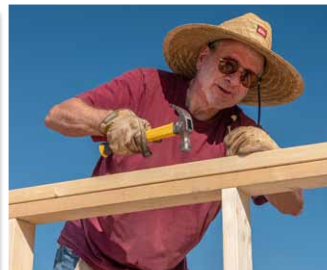
Vince Howe, above, nails top plate onto freshly raised wall section. Left: John Meyer, Dale Smith and a member of the homeowner's family steady another section of wall as it's nailed into place.
